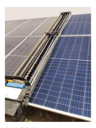
Robotic Cleaning at a plant in Rajasthan
