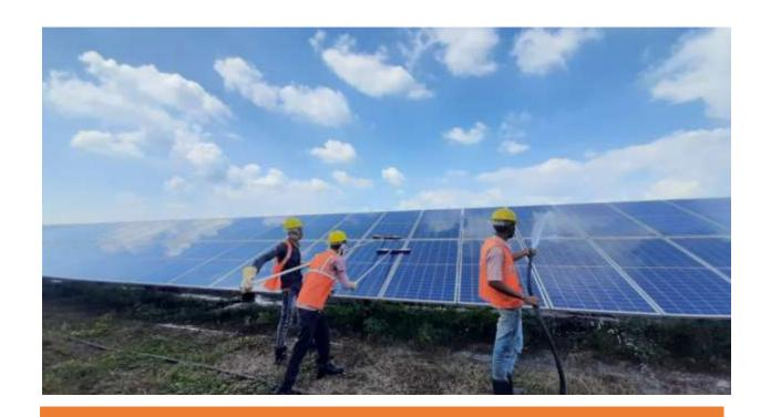
Traditional Cleaning of PV Modules using Water
